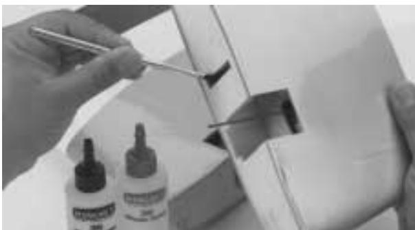
**Step 7.** Apply epoxy to the exposed portion of the wing joiner and to both wing roots.
